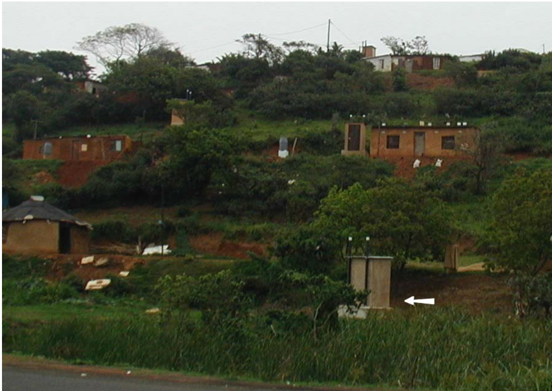
Figure 1: A double vault urine diversion latrine installed in an underdeveloped residential area
