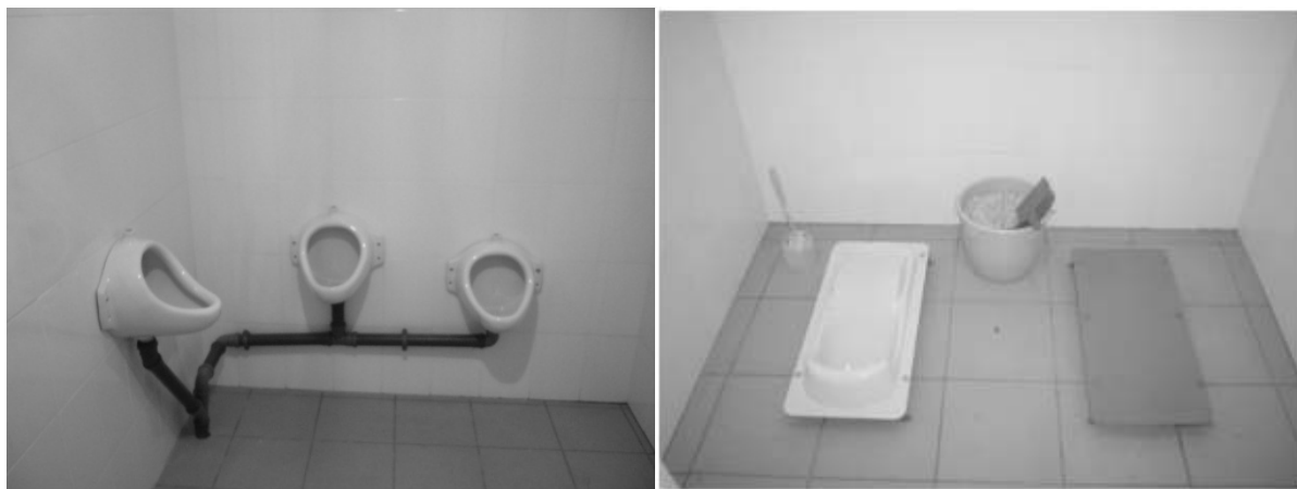
Figure 3: Inside the new school toilets
