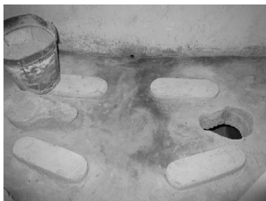
Figure 2. Ecosan squatting slab in Burkina Faso. Ashes available.
