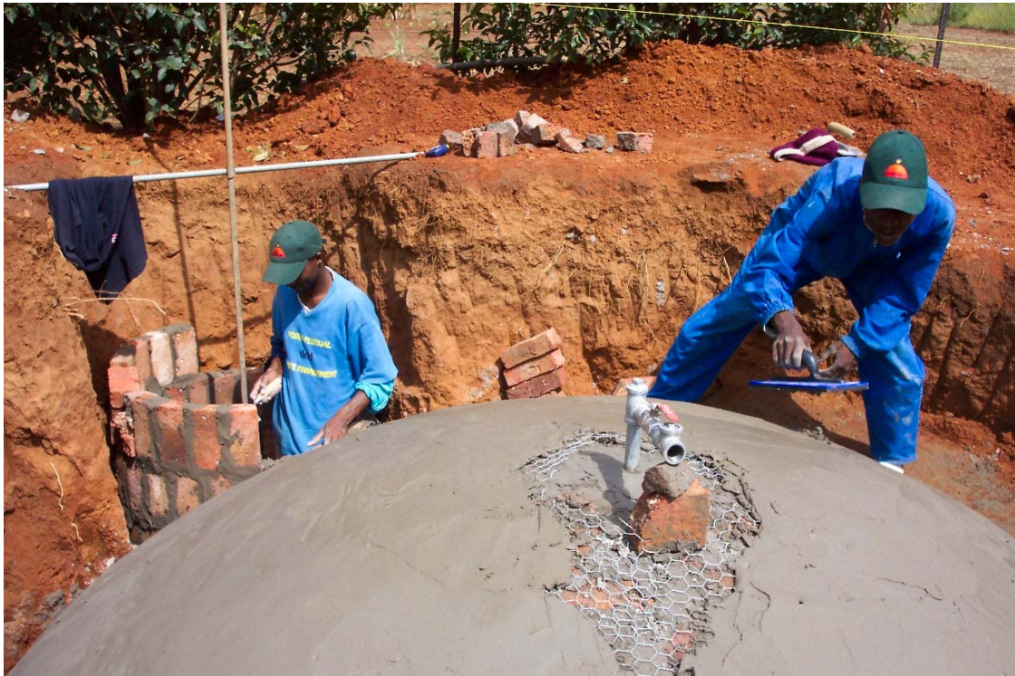
Bio-digester under construction
