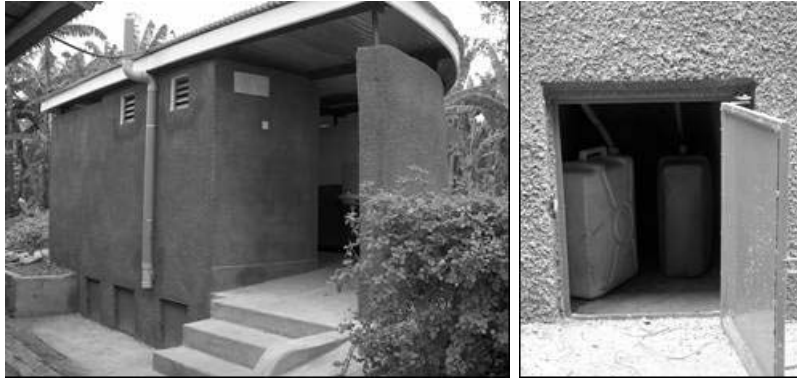
Picture 5 and 6: Demonstration Unit; Collection of urine in jerry cans
