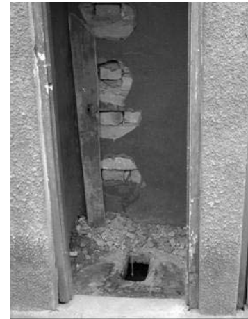
Picture 1: Pit latrine on the schools compound.
