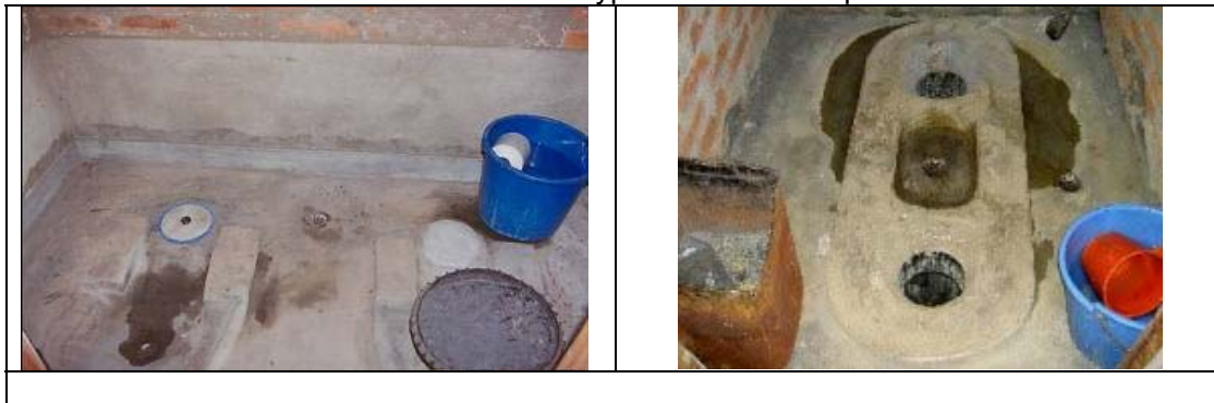
Photos 2: Different types of ECOSAN pans
